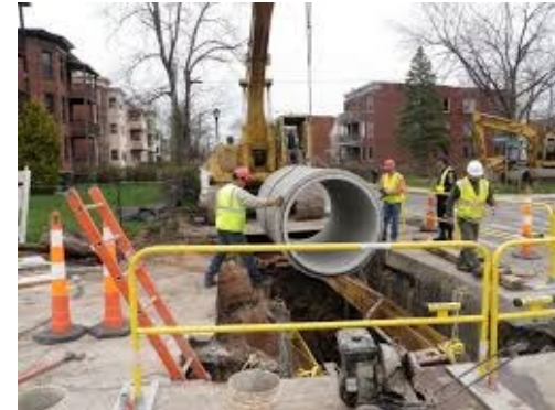
ARBORETUM SEWER PROJECT
